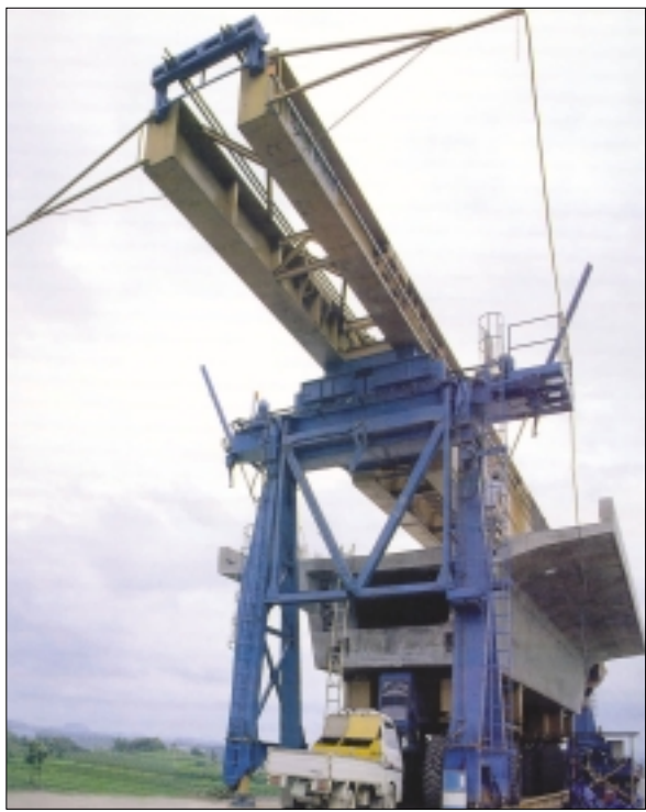
Straddle Carrier Launching Gantry
