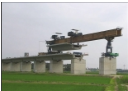
Launching Gantry 가 .
