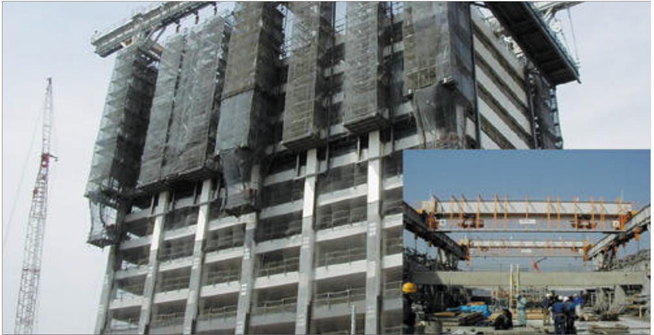
Auto-climbing Crane System [Shuttle Rise].
