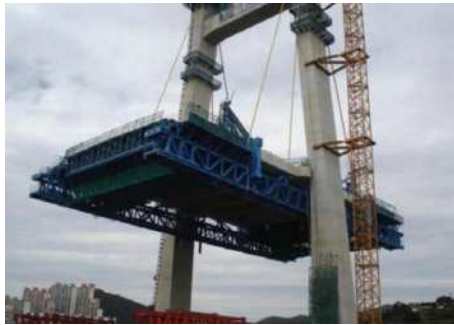
(b) F/T Heavy Lifting 완료 전경
